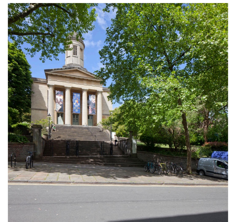
Fig: 199 Existing view
