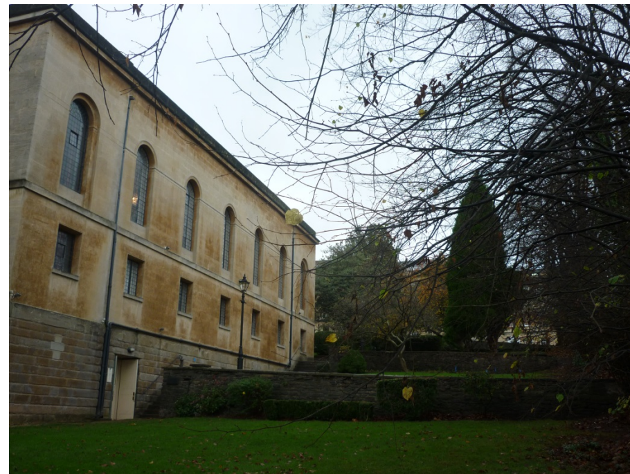
View from within the site looking West
