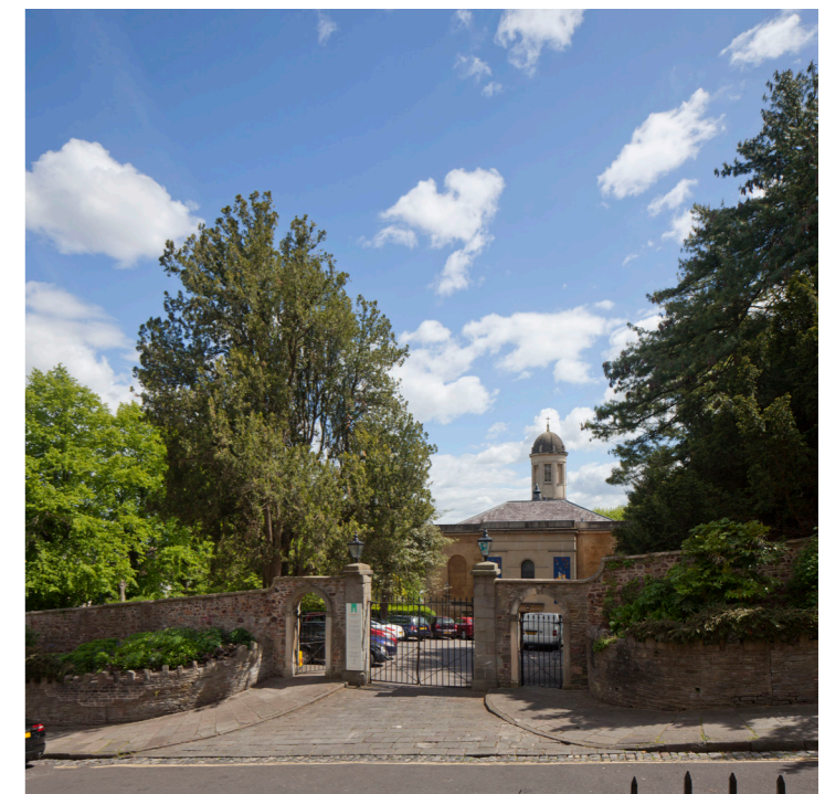
Fig: 203 Existing view
